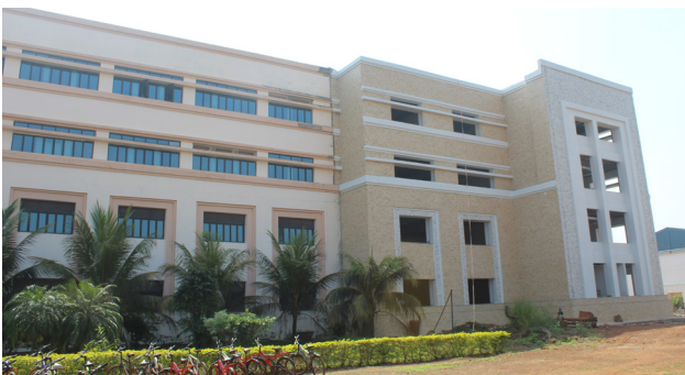
SMS Extension Building
