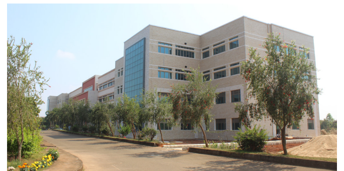
SES Extension Building
